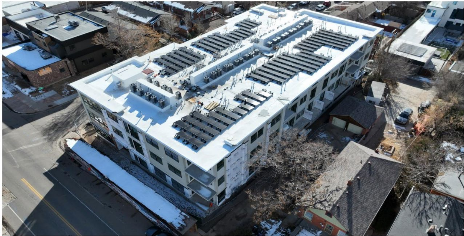
NW Corner-Facing SE
