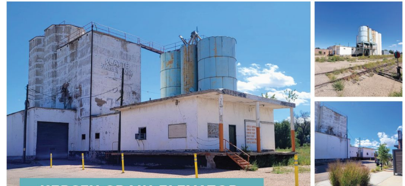
KERSEY GRAIN ELEVATOR
