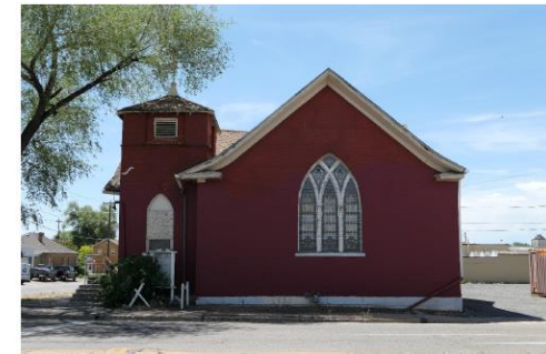
Photo 2: North side. Camera facing south.
